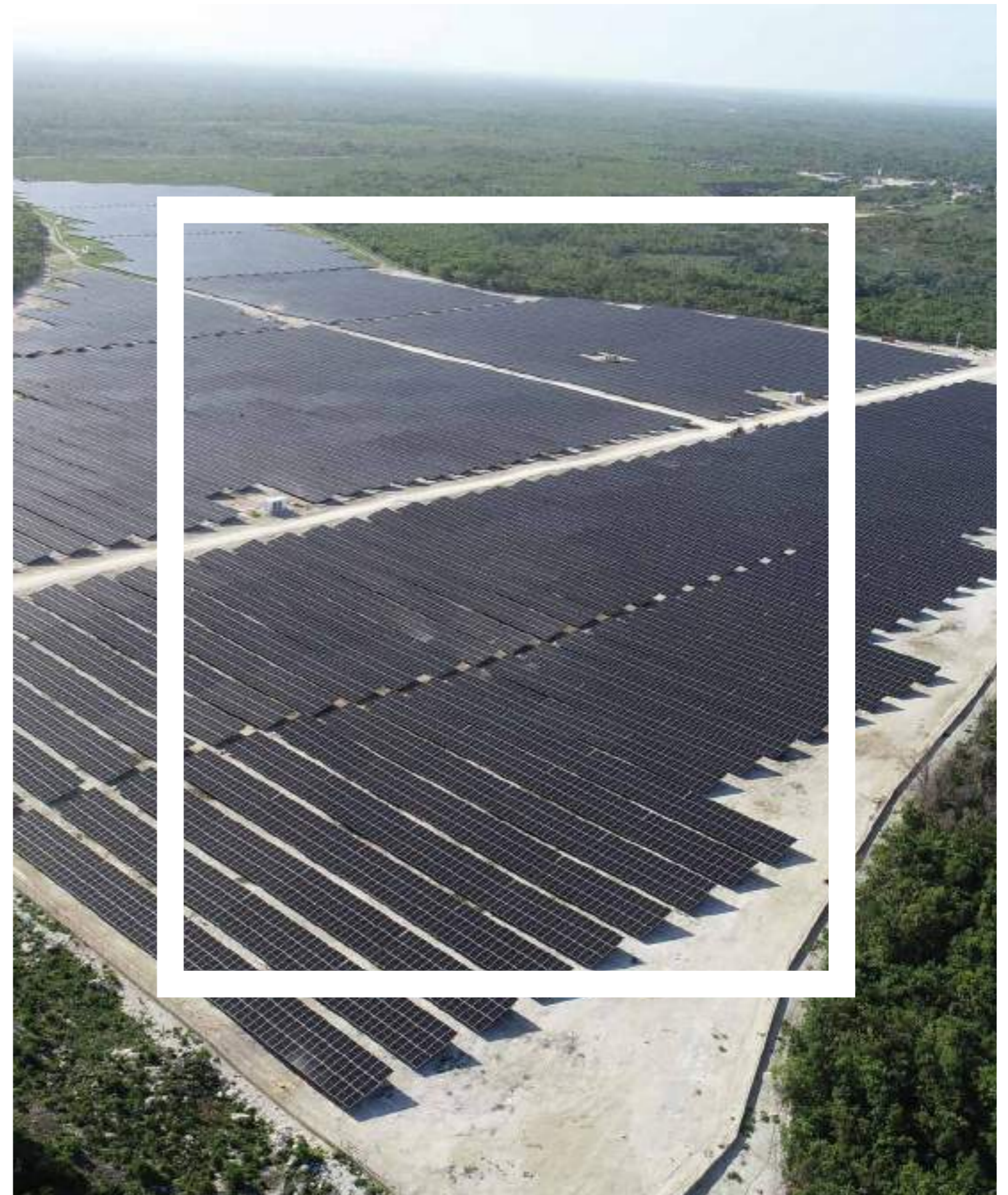
Bávaro solar photovoltaic power plant (Dominican Republic)
