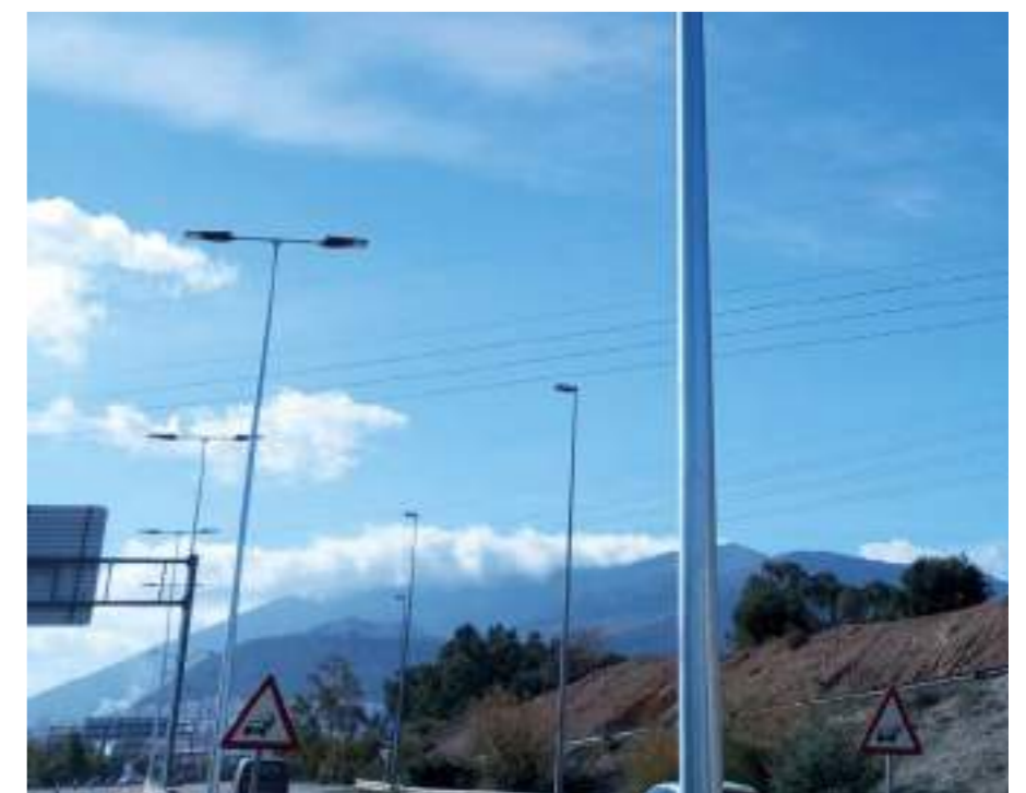
Public lighting on roads, Jaén (Spain)
