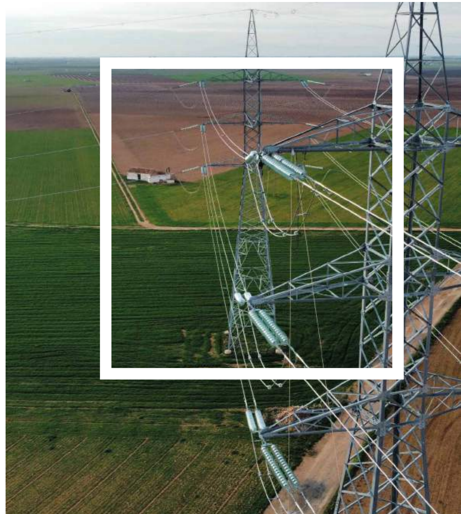
Insulator replacement on the evacuation line of the Nudo Manzanares SET (Spain)
