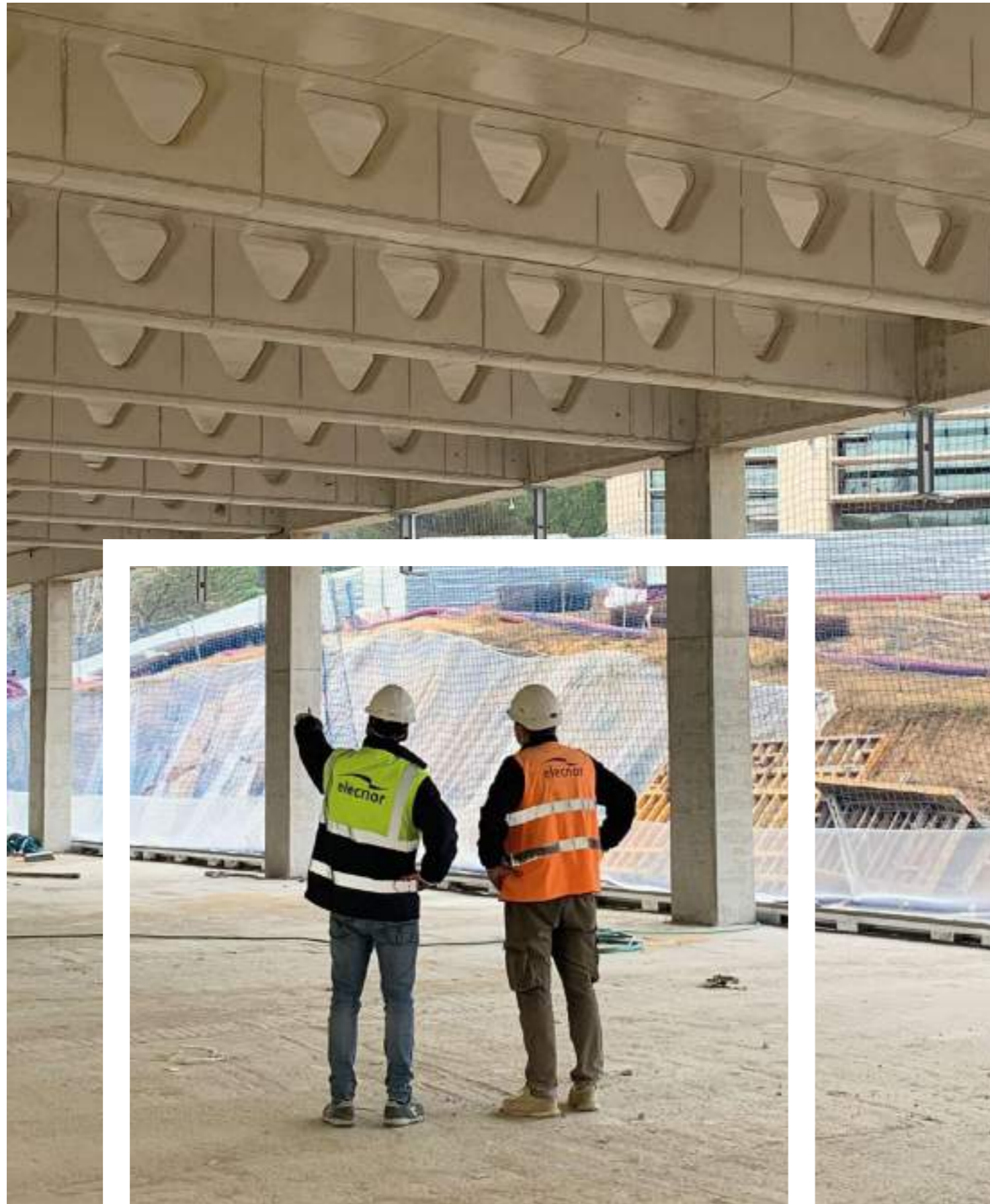
Construction and installations of offices for Nosce Roche, Barcelona (Spain)
