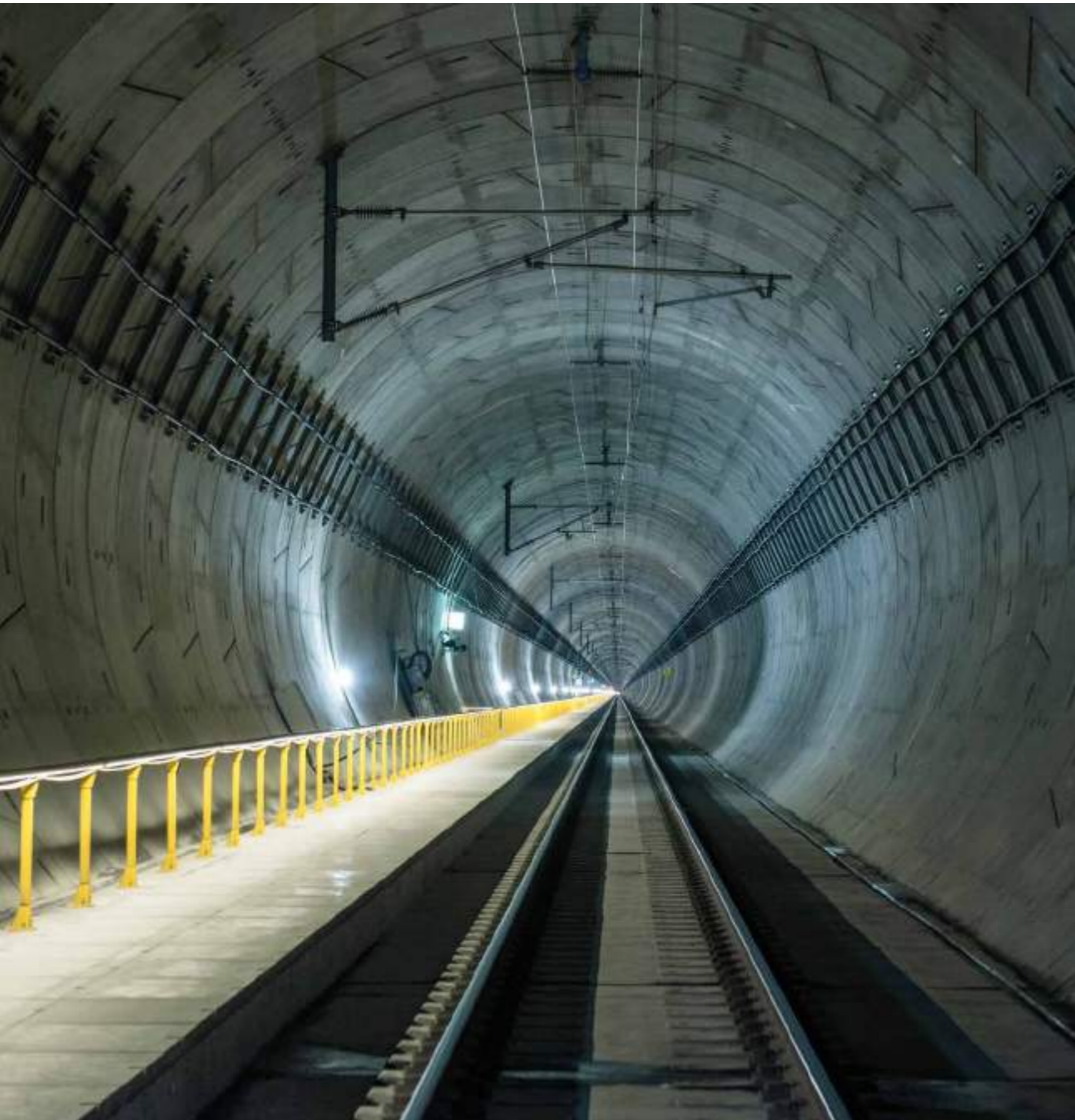
Follo Line project (Norway)
