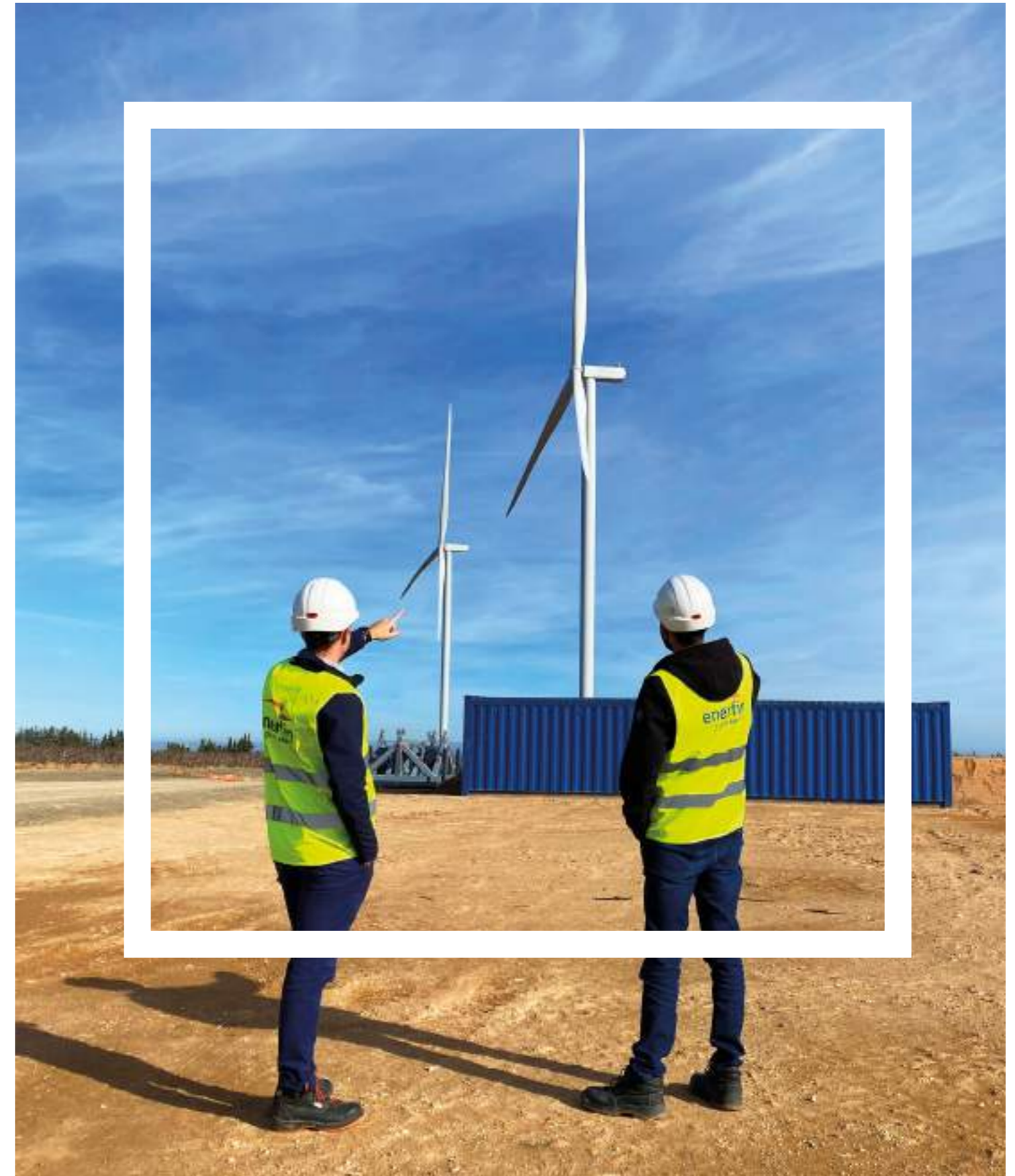
Renovables del Cierzo Wind Power Complex in Navarre (Spain). Enerfín
