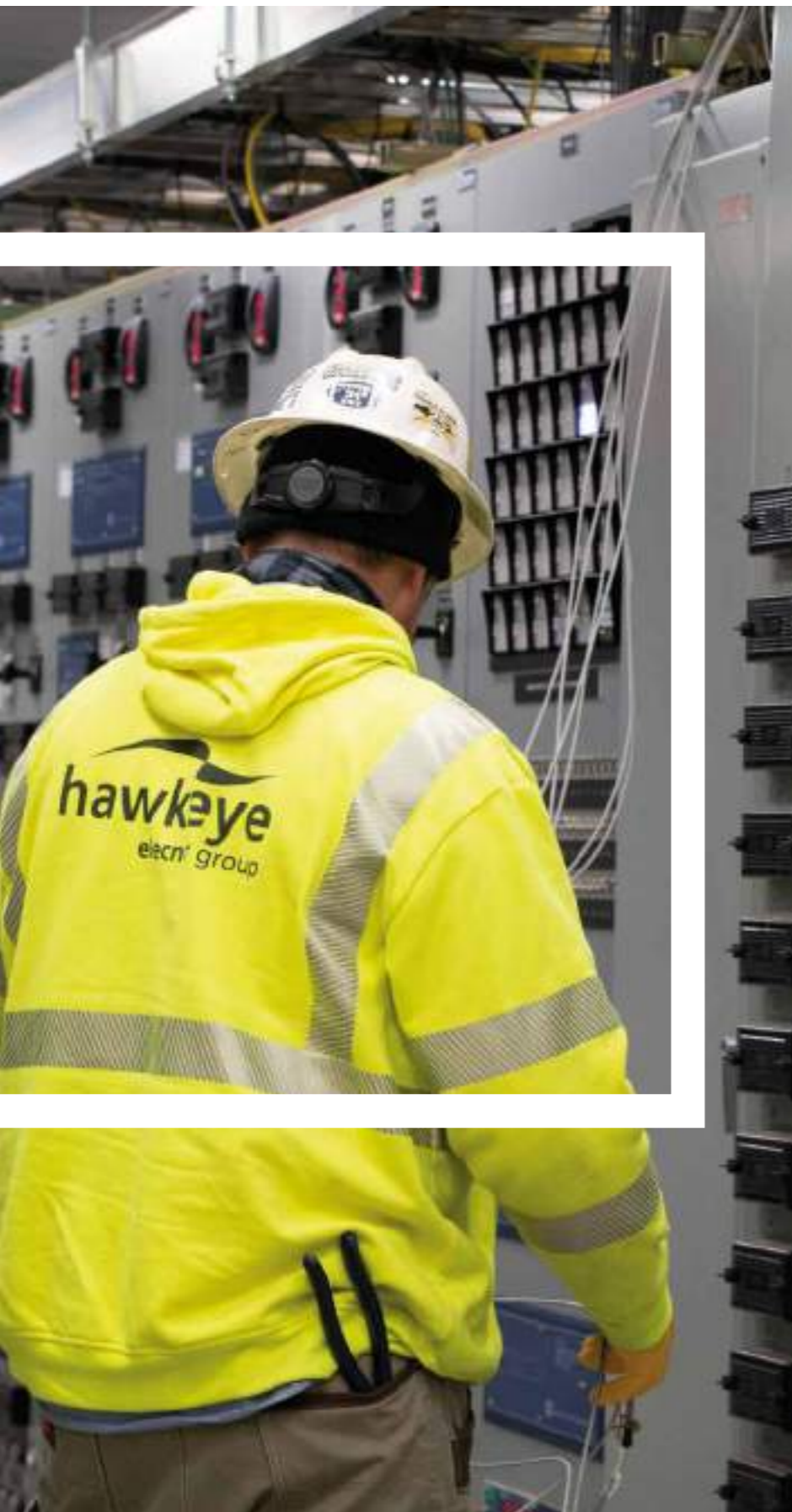
Substation expansion at Riverhead, New York (United States). Elecnr Hawkeye
