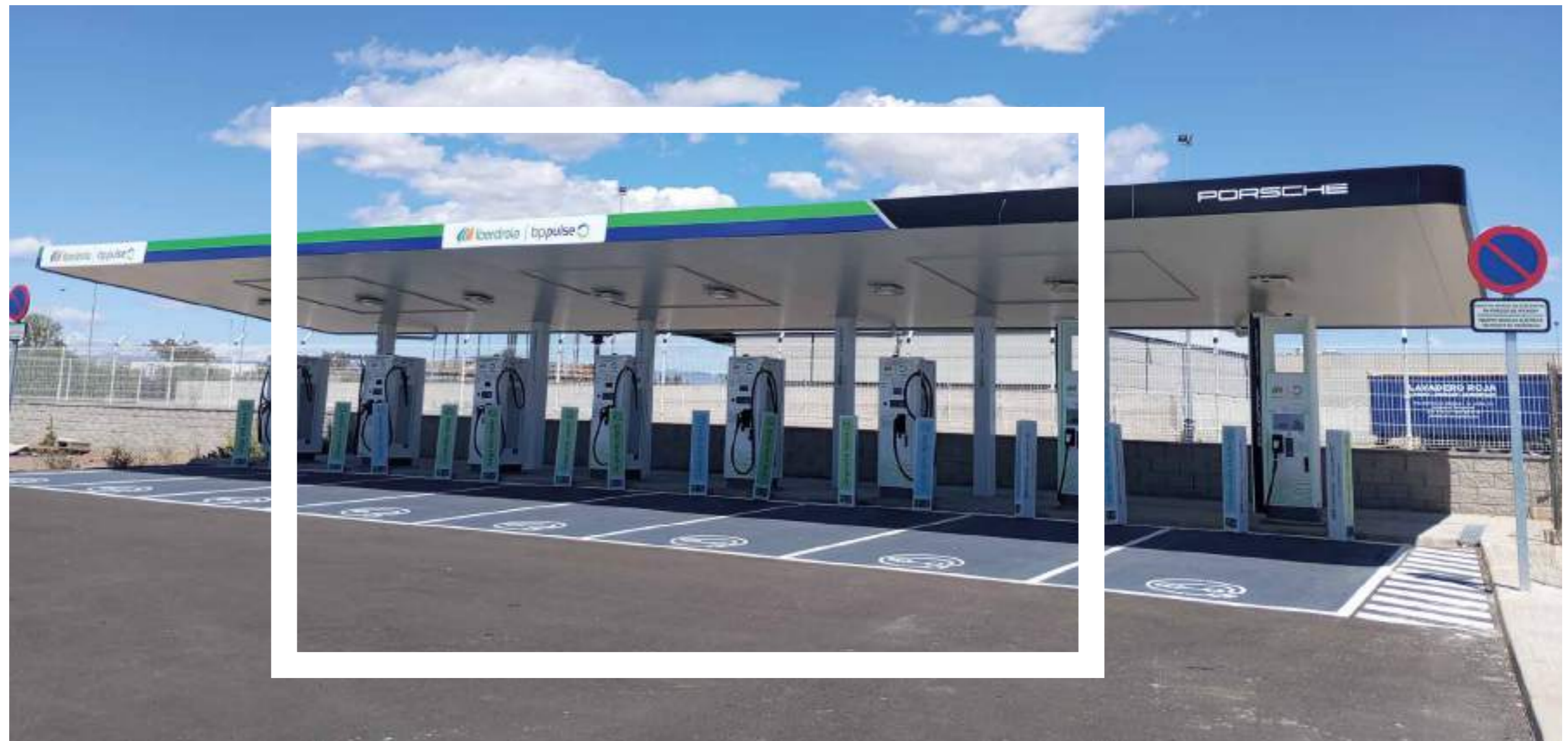
Porsche-Iberdrola charging point, Castellón (Spain)
