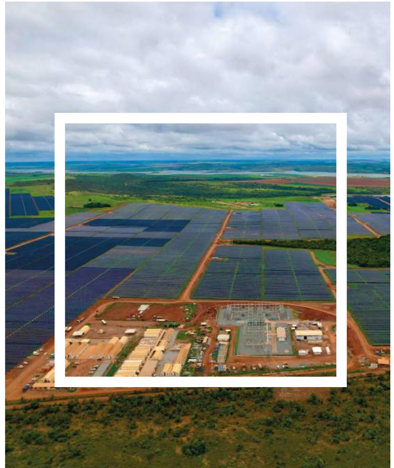
Boa Sorte solar photovoltaic power plant (Brazil)
