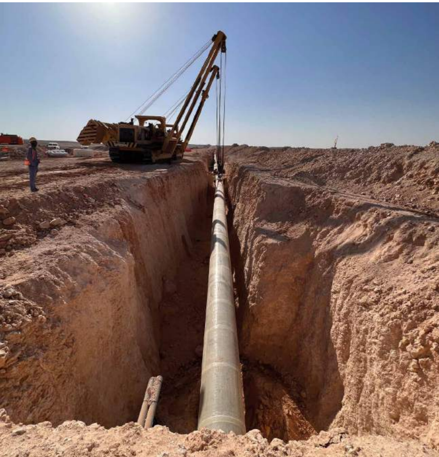
Salalah gas pipeline (Oman)
