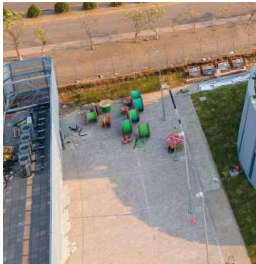
Palmerola International Airport (Honduras)
