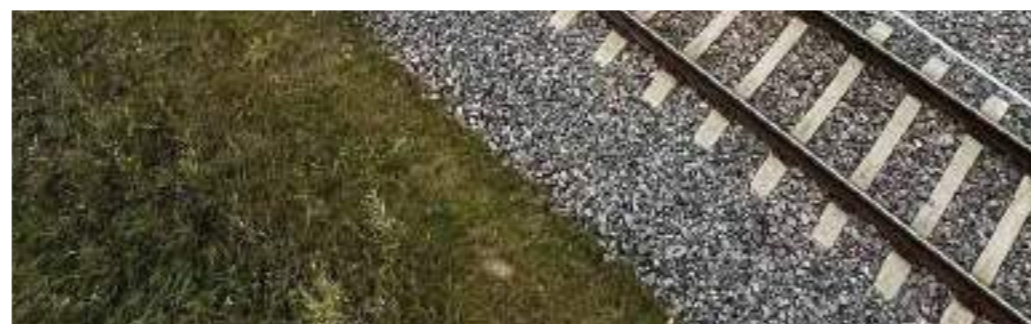
Vilnius-Kapleida railway electrification (Lithuania)
