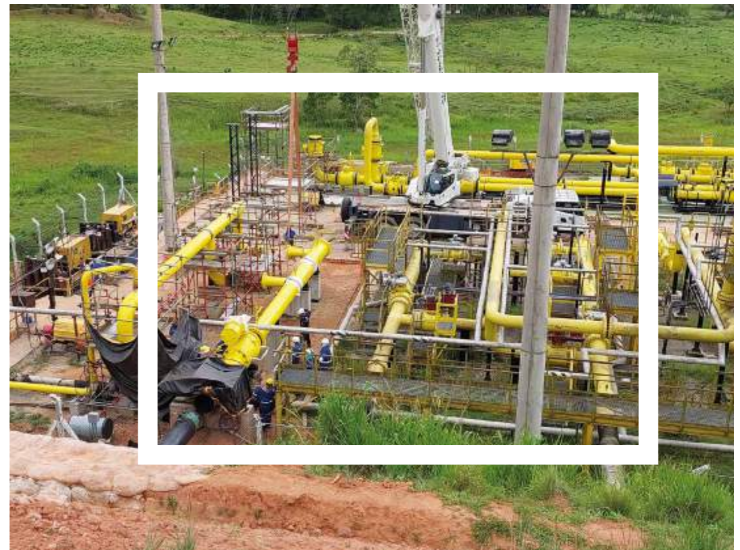
Gasig gas pipeline (Brazil)
