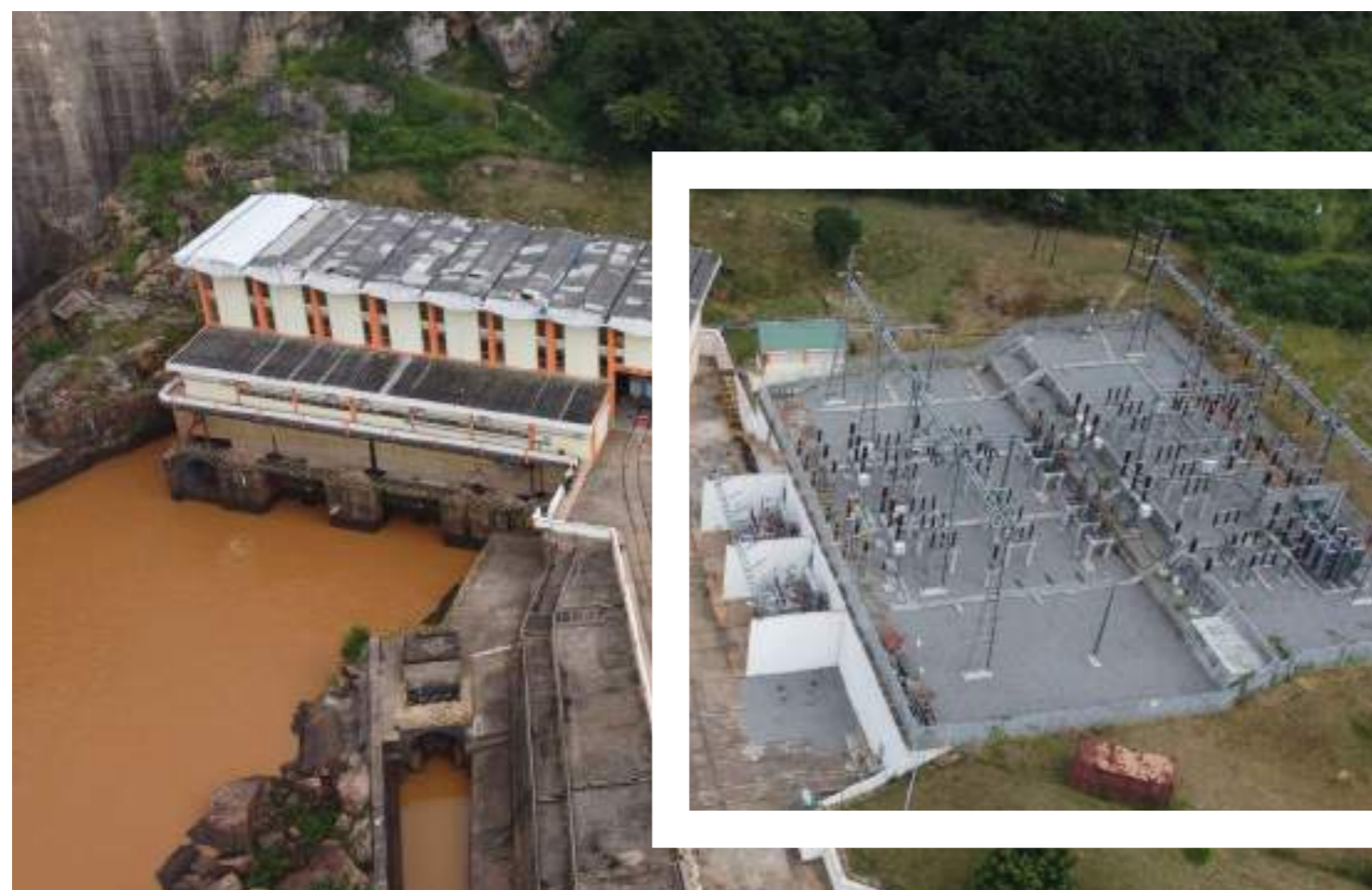
Chicamba Hydroelectric Power Plant (Mozambique)
