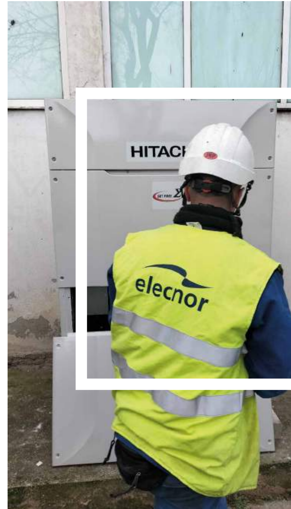
Air conditioning installation at Renault, Seville (Spain)
